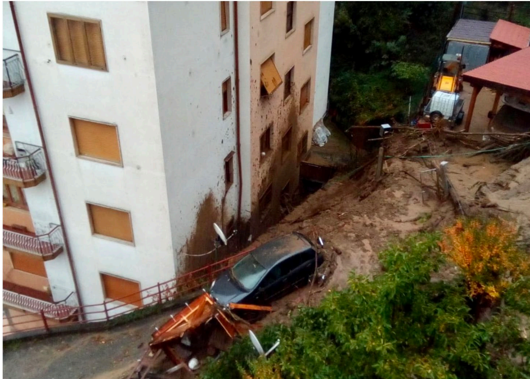
Heavy rain triggered landslides in northern Italy, 20 to 22 October 2019. Photo: Vigili del Fuoco
