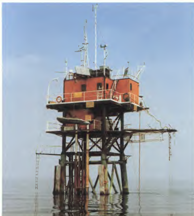
The CNR Oceanographic Research Platform off the Italian coast, near Venice. The upper decks of the tower have since been modified to accommodate a PRARE station and microwave radiometer.
