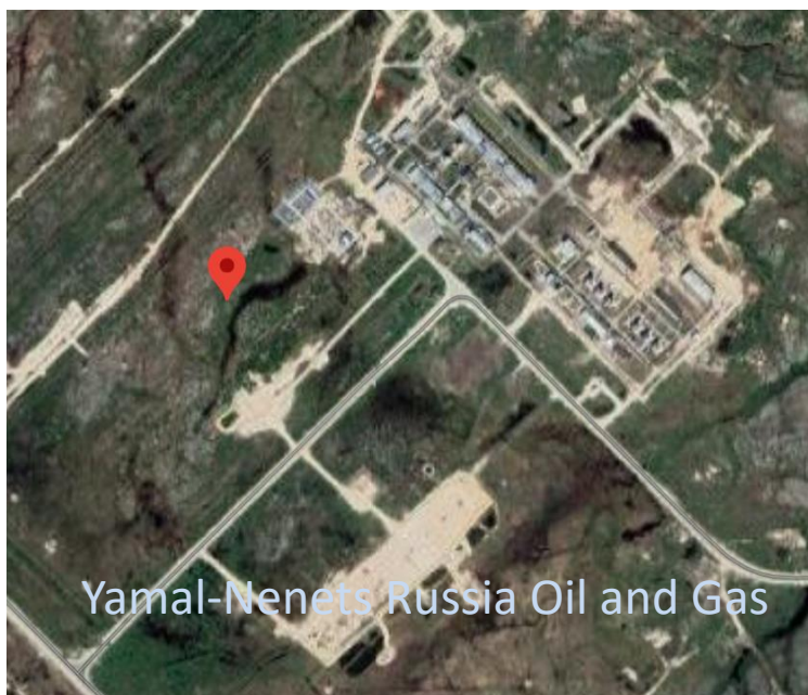
Figure 15 – Russia, Oil and Gas Yamal-Nenets Infrastructure site
