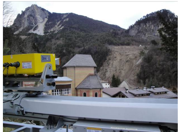
Figure 11. Picture of the Perarolo di Cadore landslide monitoring site.
