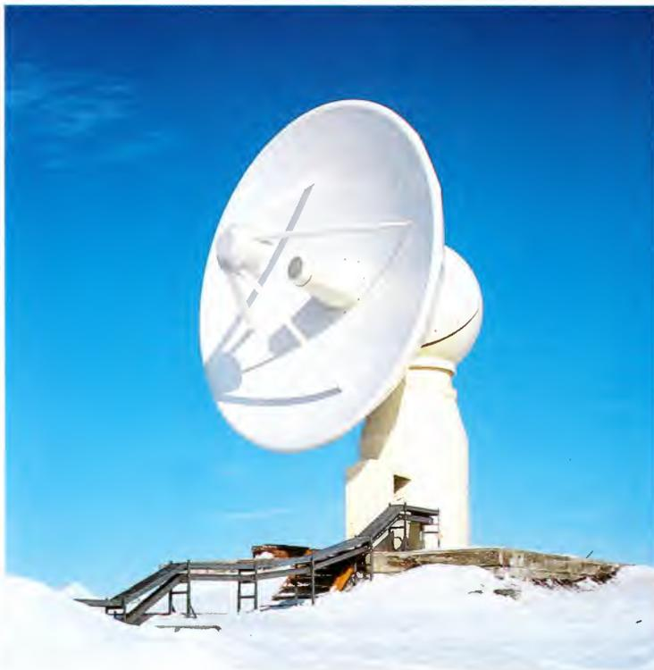
The photo above shows the German ERS-1 ground station in Antarctica, although "ice station" would be a more appropriate description. ERS-1's radar coverage would not be complete if it did not include the sixth continent, where the wind often exceeds 200 kph and temperatures can drop to  $-70^{\circ}\text{C}$ .
