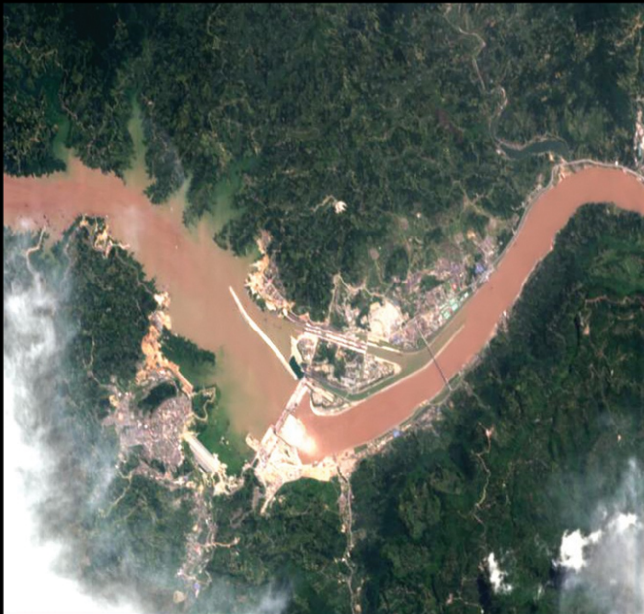
Three Gorges Dam, China
