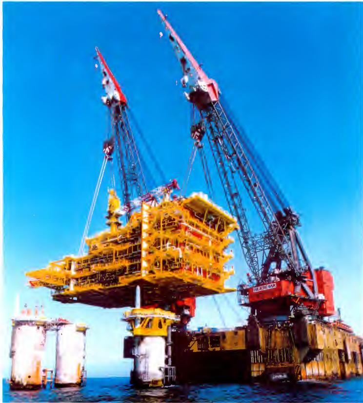
Crane barge hoisting drilling and accommodation facilities into place
