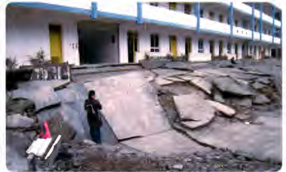
↑ A school located on the Wenchuan earthquake fault. The girl in the foreground stands next to the fault scarp. Courtesy of Xu Xiwei and Yang Hu (IGCEA).
